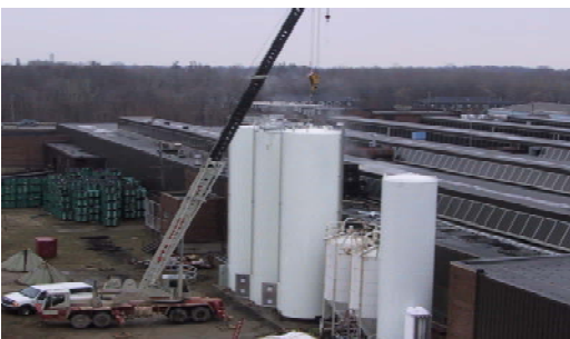
Silos being installed by Eagle Installation Crew on Load Stands
