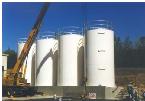
Welded Smooth-Wall Steel Tanks
