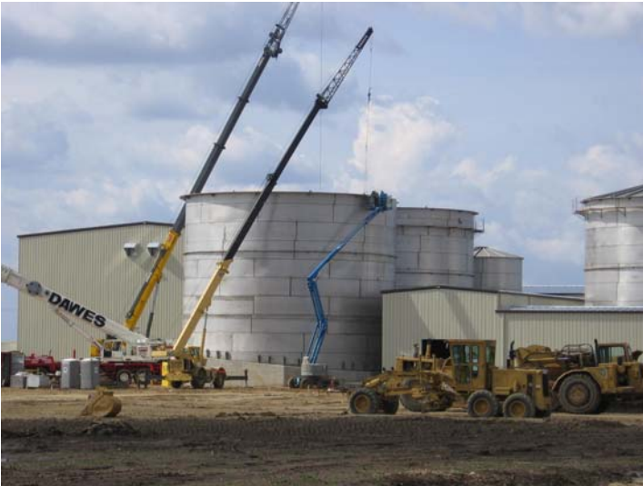
Field Welded Tanks Installation on Foundations by Eagle Install Crews
