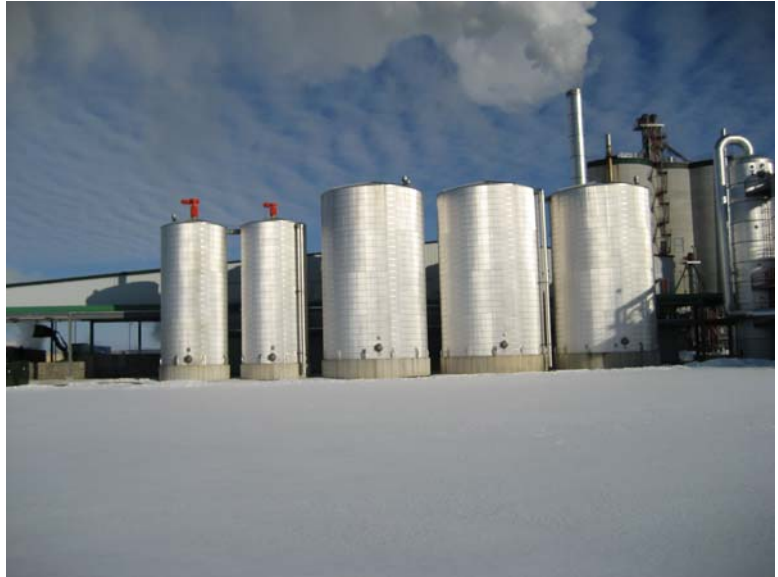
Field Welded Tanks Installed Complete on Foundations
