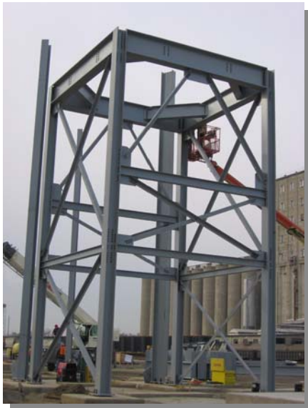
Custom Fabricated Tank Structure being installed by Eagle Install Crews.
